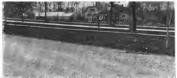
ANOTHER SECTION OF SAME ROAD NOT TREATED WITH TARVIA.
